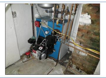
**2.0** The heating system was shut down at the time of this inspection, the oil tank was empty, and having the system turned on prior to the final walk through to verify proper operation is needed. The boiler T / P relief valve extension tube is missing and the installation of one is needed for safety.
