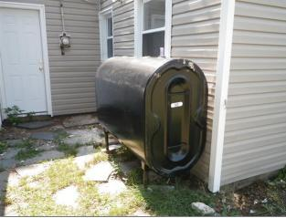
**2.1** The oil tank is being supported in an unconventional and unsafe manner and the installation of a concrete pad by a qualified contractor is needed for safety. The oil tank fill and vent ports are not installed, the tank is empty, the oil tank has been installed in front of a window, and relocation / repairs by a qualified contractor are needed. The home contained a prior underground oil tank and obtaining all documentation associated with the oil tank abatement is recommended.
